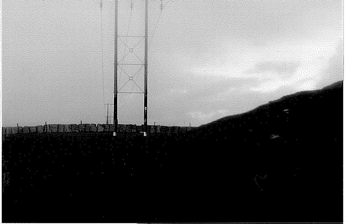
Pole 131 View from SE Broch on immediate right.
