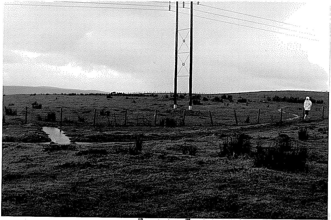
Pole 105 View from East Enclosure in foreground
