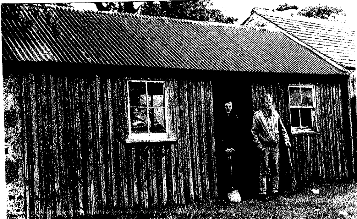
'HOME GUARD' HUT BEFORE RENOVATION
