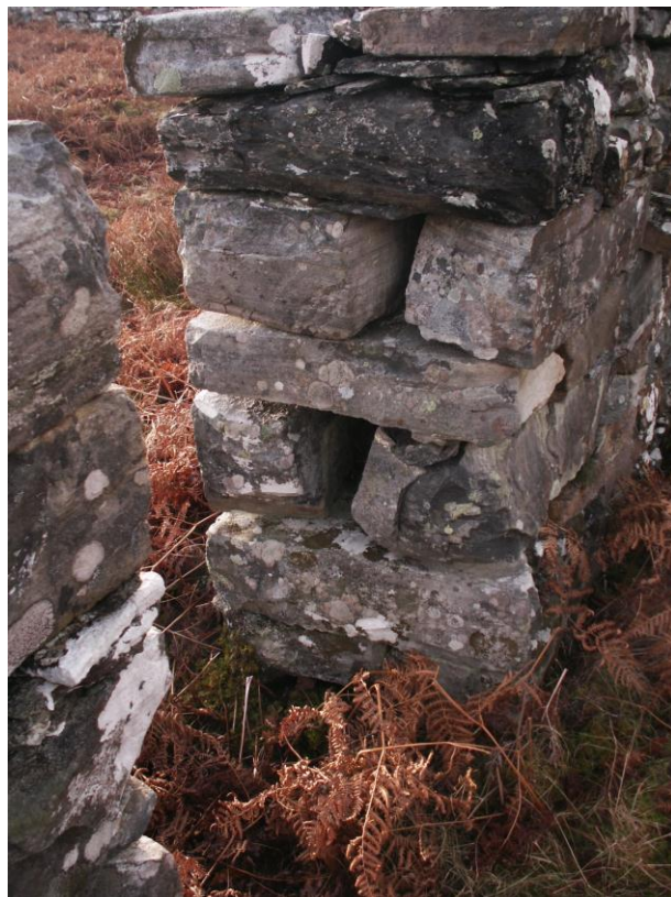
Slots in doorway of main building
