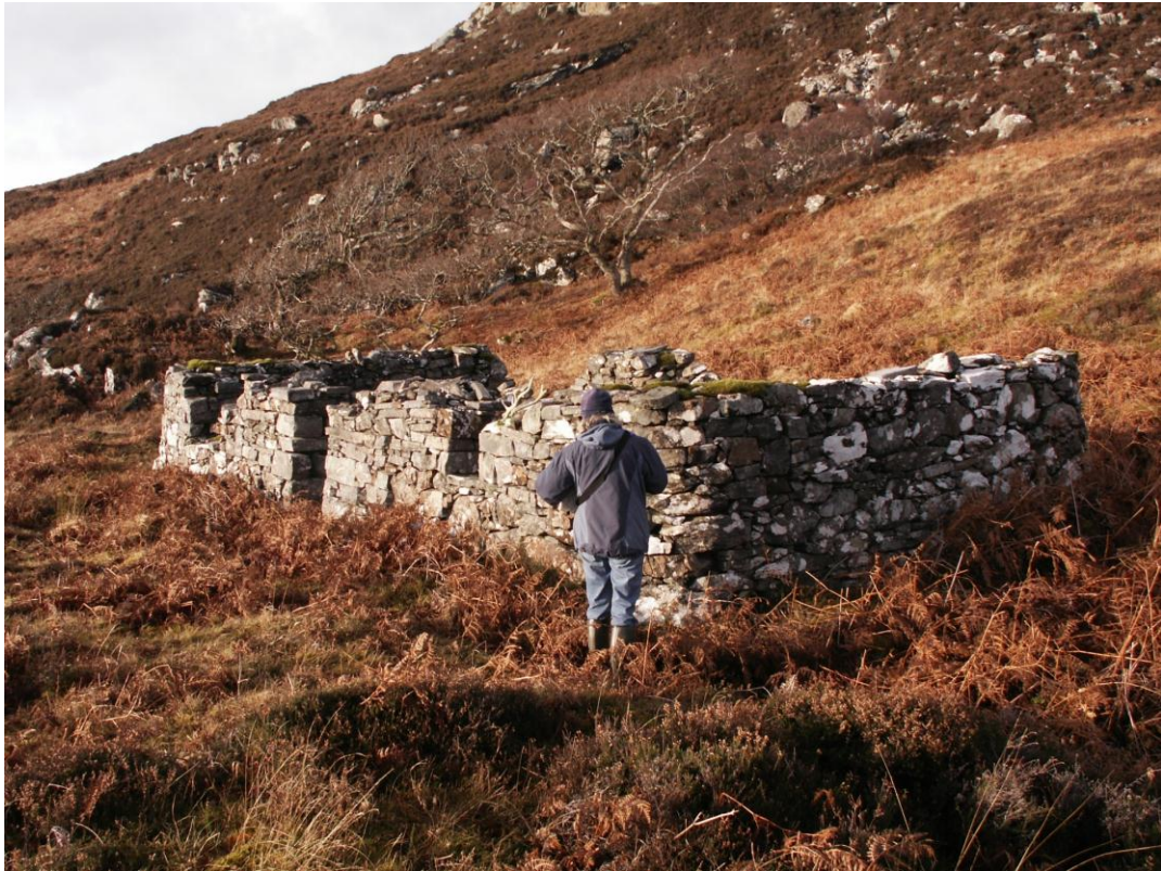
Main (north) building
