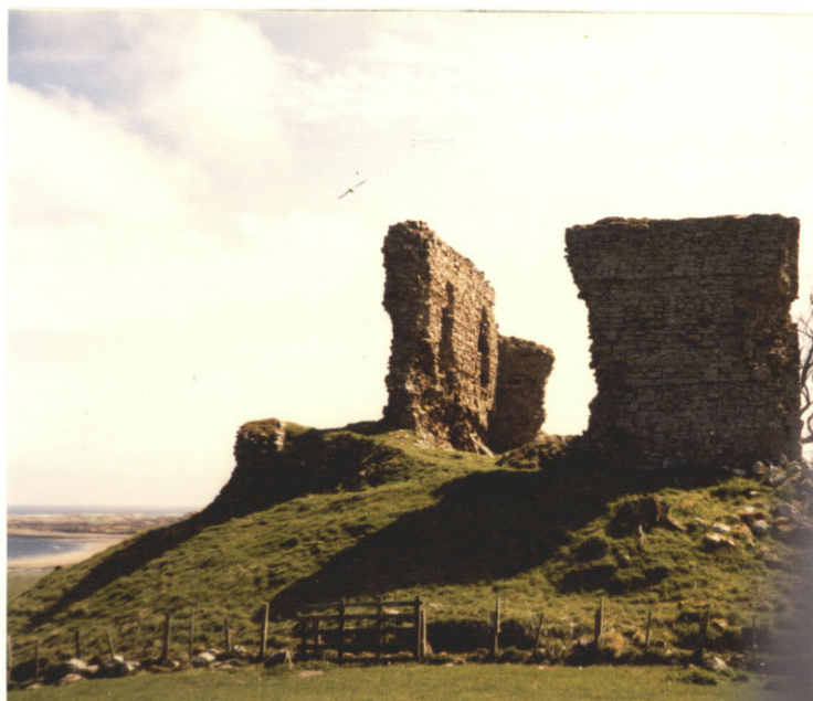
NE and NW facing walls and summit of knoll taken from WNW.
