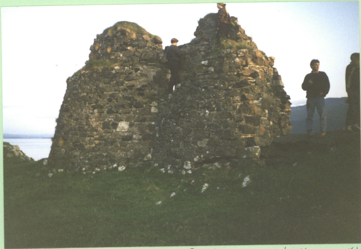
NM 64 SE 001 Ardornish Castle interior looking south at reconstruction work from 1910s. during SOMAP94 visit Aug 1994.
